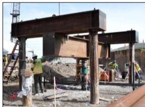
Static Load Test
